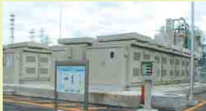
▲ NaS Battery in Sunamachi WRC
