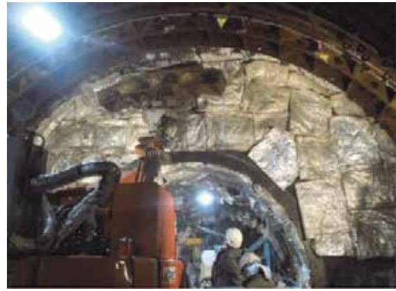
Fig.13 Segment assembling
