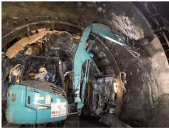
Fig.12 Frozen soil drilling
